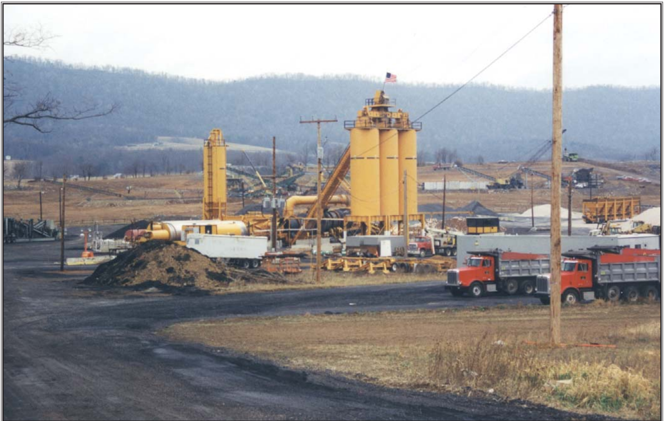
A modern HMA facility provides high production, good quality mixes (including recycled asphalt pavement if desired) while meeting stringent air quality standards.
